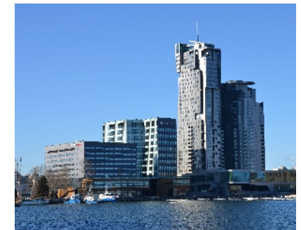
Sea Towers Gdynia
